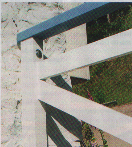
▲ Fixing to the wall by 200mm screws...
