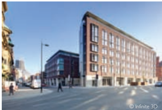
The height of the building at the front was reduced to stop it being too overpowering and the repeated window openings are in proportion to neighbouring buildings. Note the closeness of Liverpool Metropolitan Cathedral
