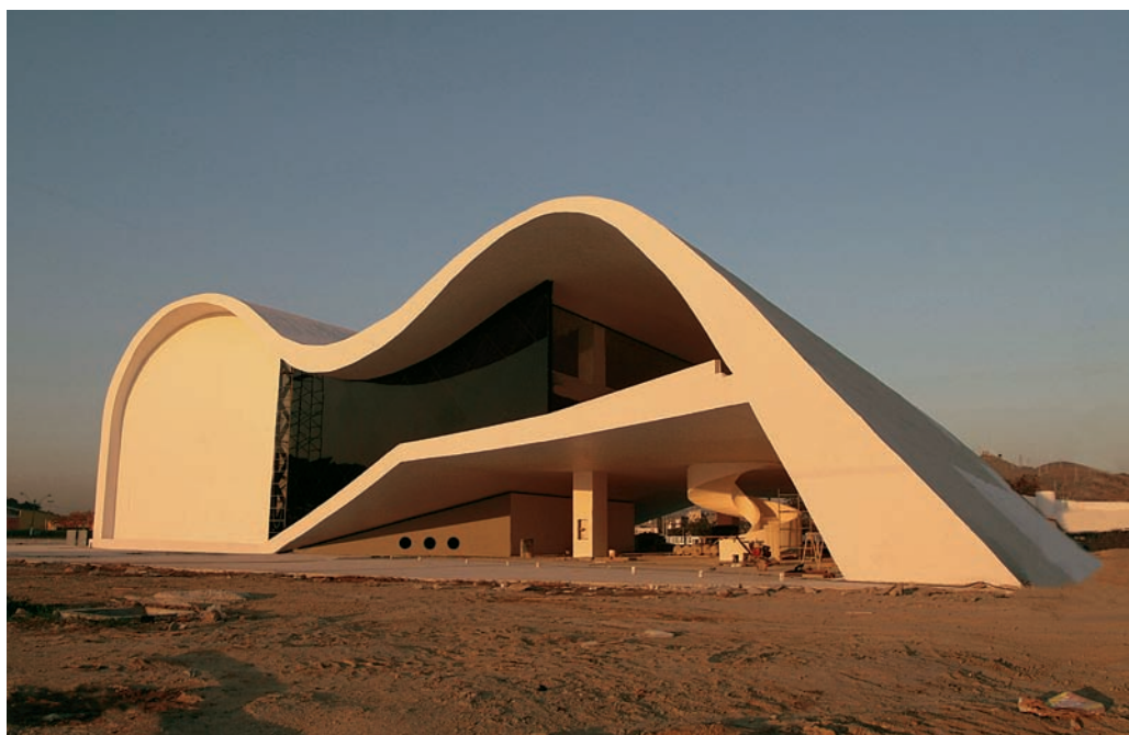
Left and below the planning and construction phases of the National Theatre, which opened last month and which will form part of a complex of cultural buildings at Niterói
