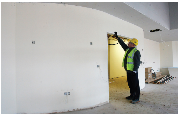
A contractor examines a wall plastered using Knauf MP75 projection plaster
