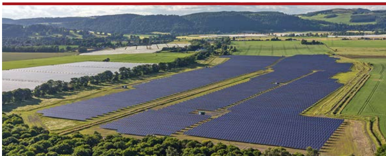
ARRAY OF SUNSHINE: Elgin Energy completed the 13MW Errol near Perth, Scotland's largest solar farm, in 2016. The company secured permission last year to build the 50MW Milltown Airfield farm in Moray, which would be the most northerly in Scotland. Photo: Elgin Energy
