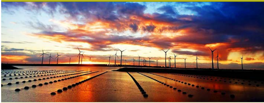
PARALLEL PARKING: Deltawind has completed construction of its 102MW Krammer wind farm, featuring 34 Enercon E-115 3MW turbines with 180-metre tips, in the Dutch province of Zeeland
