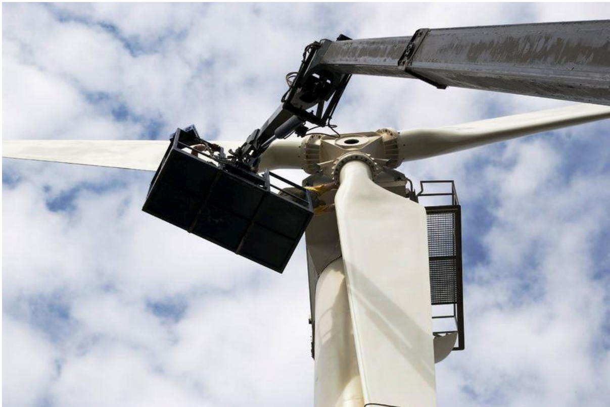
Image Wind turbine decommissioning
